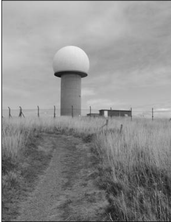
A modern radar now stands at a corner of the former RAF site.
