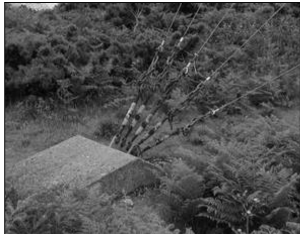
An aerial halyard anchor block. The illustration below (of a modern communications mast) demonstrates how halyards are anchored.
