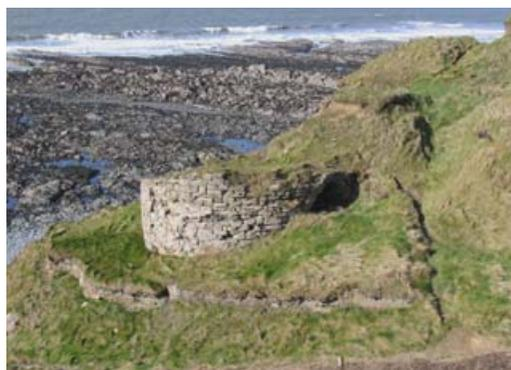
Limestone, brought by boat from South Wales, was loaded into the kiln from the top, interspersed with layers of coal. Burnt slowly, it produced powdered white lime for fertilizer and it was also used in limewash paint, and lime mortar.
