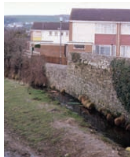
THE OLD SEA WALL AT WRAFTON
